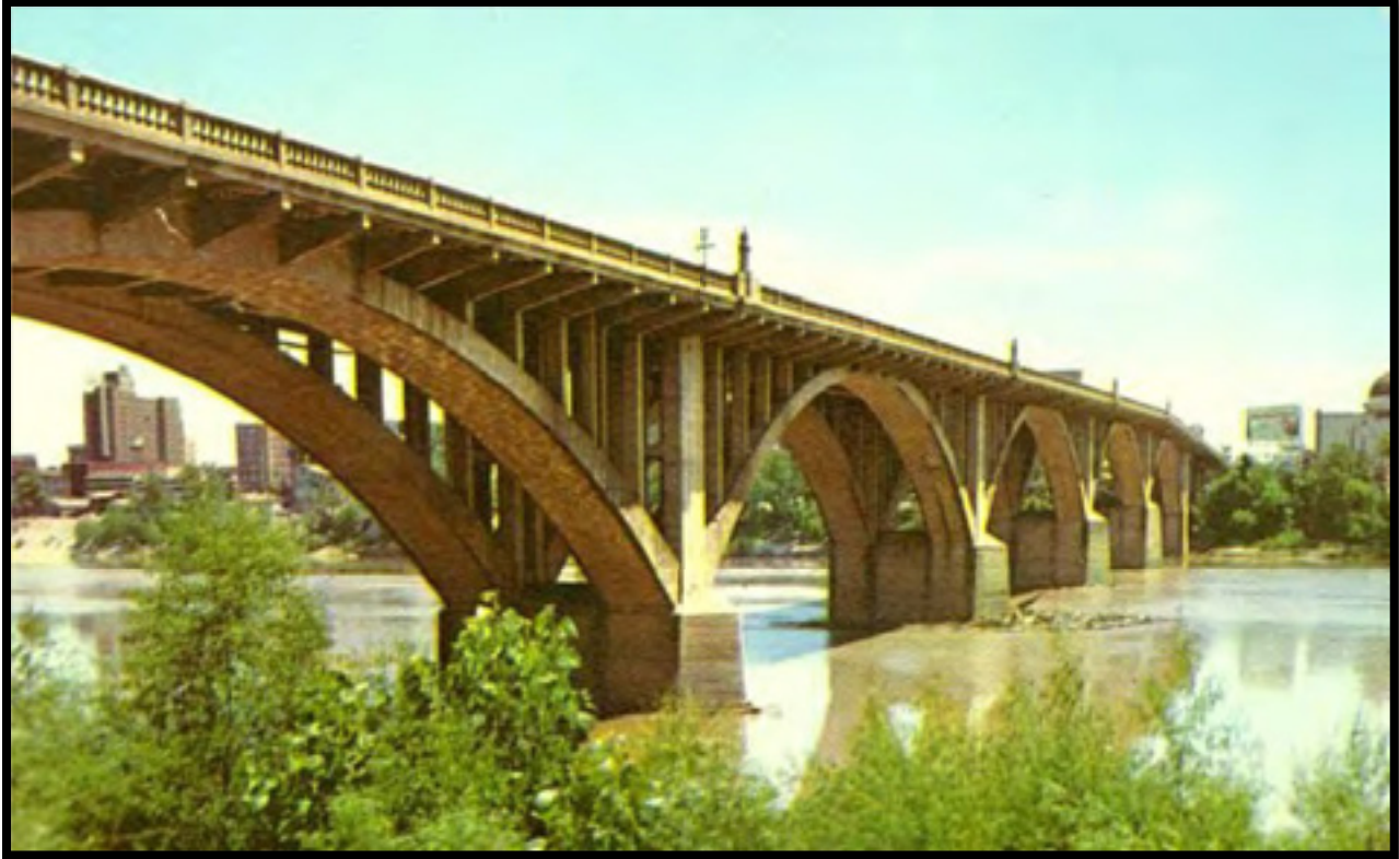
Figure 32. Broadway Bridge (circa 1968)
