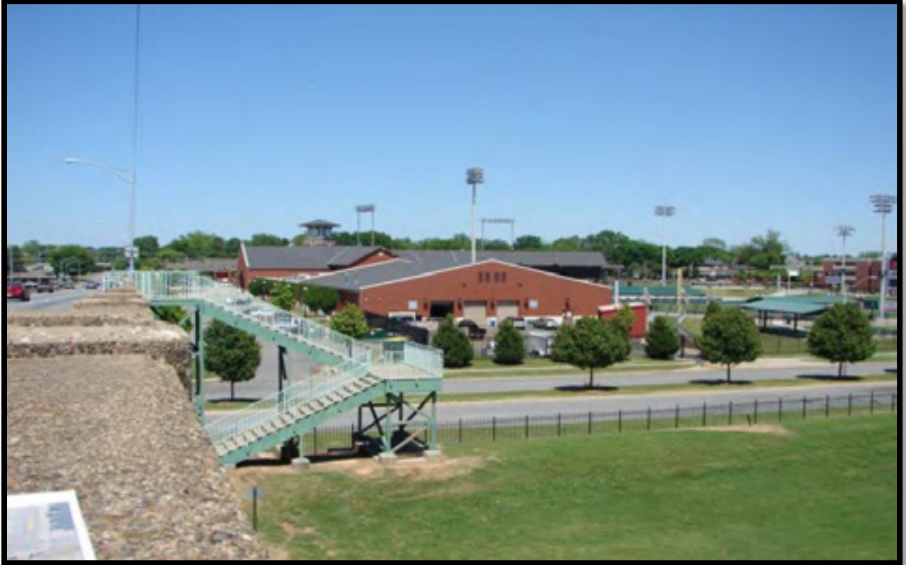
Figure 25. Stair access to NLR's Riverfront Park
