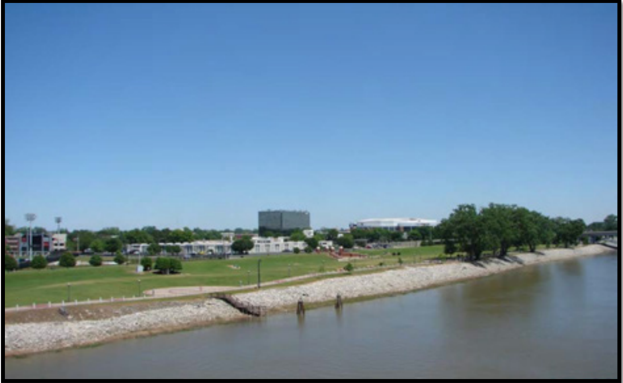
Figure 19. View to the northeast from the Broadway Bridge
